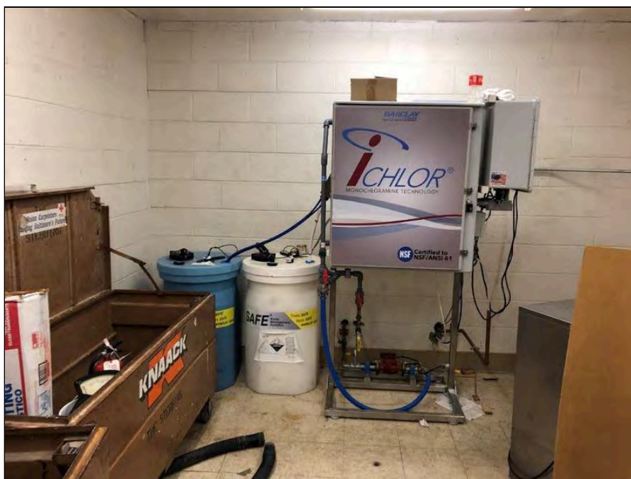
12 - Representative water treatment system
