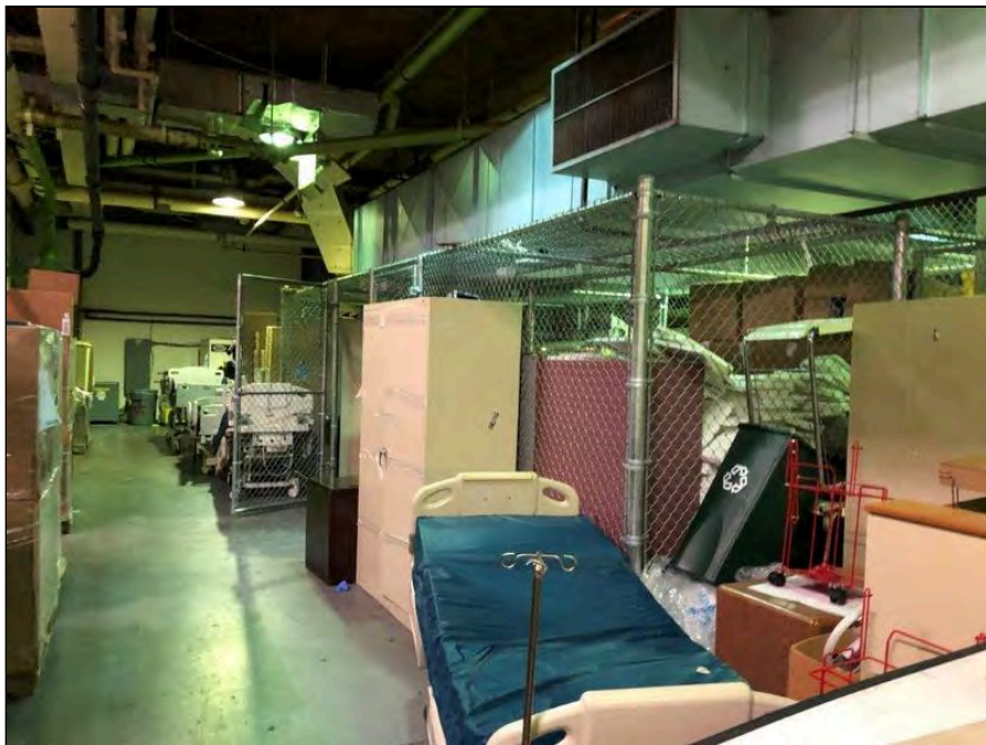
14 - Hospital basement storage, facilities offices
