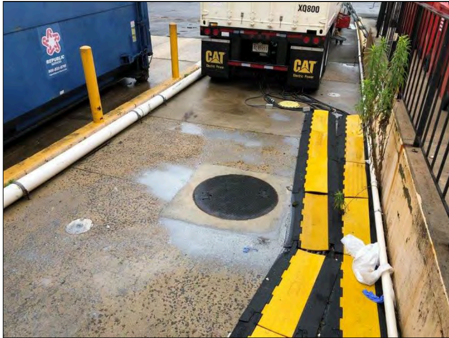
27 - Suspect 5,000-gallon diesel fuel UST
