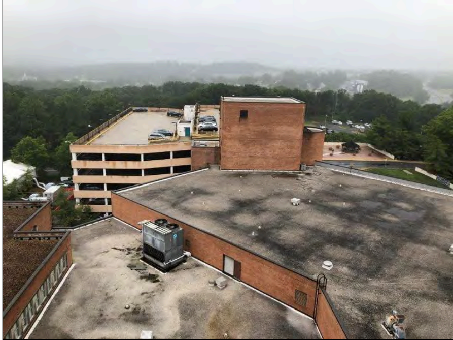
23 - On-site structure, parking garage
