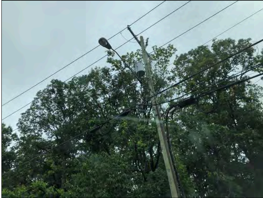
43 - Pole-mounted transformer
