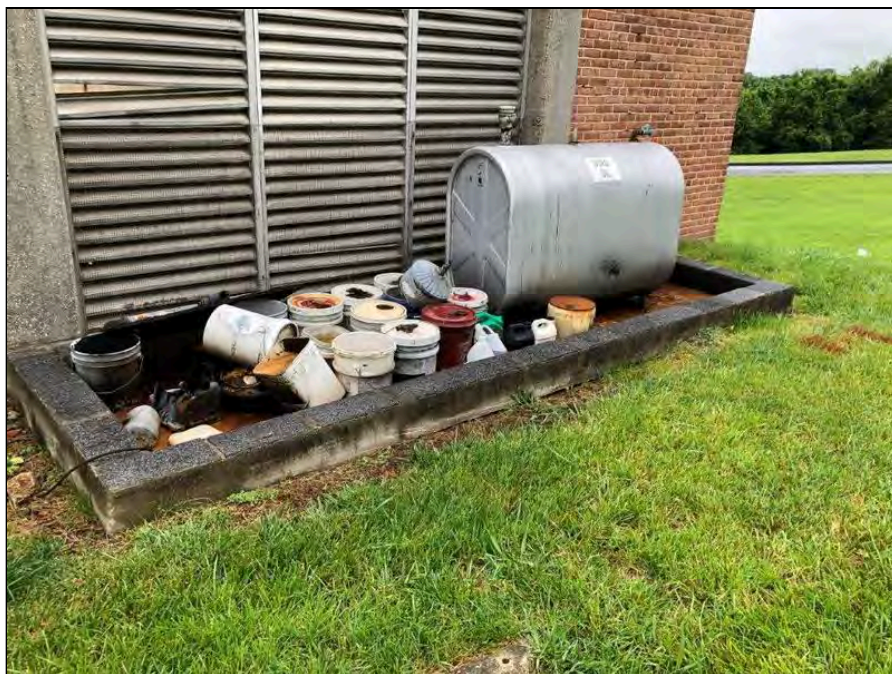
21 - 275-gallon used oil AST, leaking 5-gallon bucket containment
