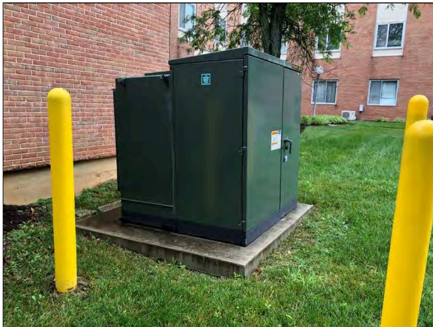
28 - Pad-mounted transformer
