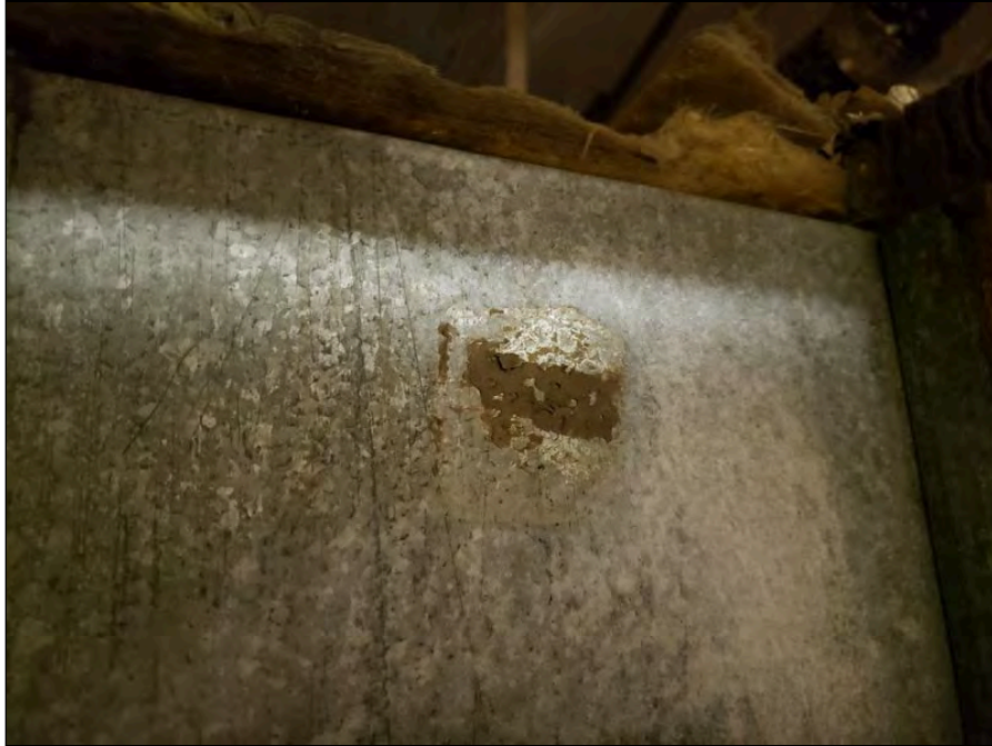
11 - Duct Pin Mastic (ACM)
