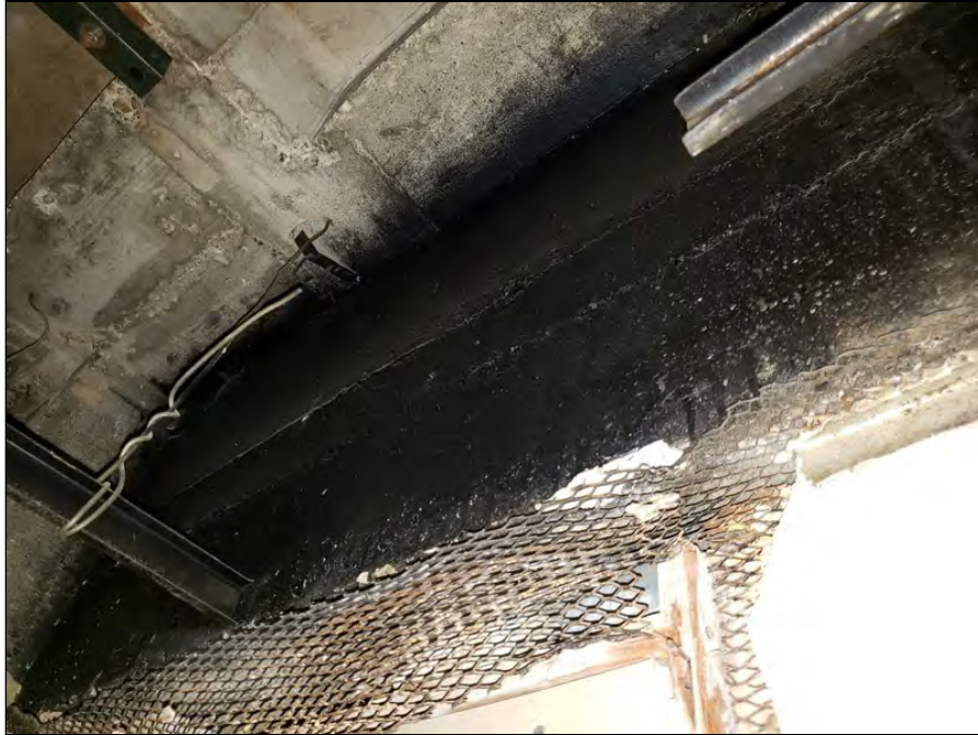
3 - Black Waterproofing (ACM)
