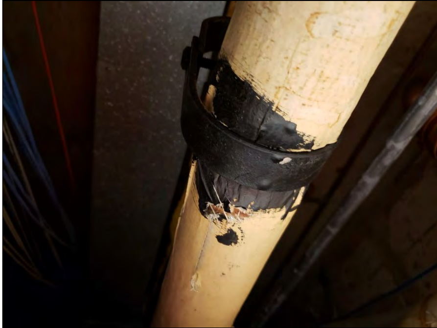
1 - Black Thermal System Insulation Hangar Mastic (ACM)
