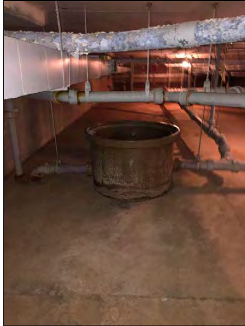
13 - Former chemical storage pool in the basement crawlspace
