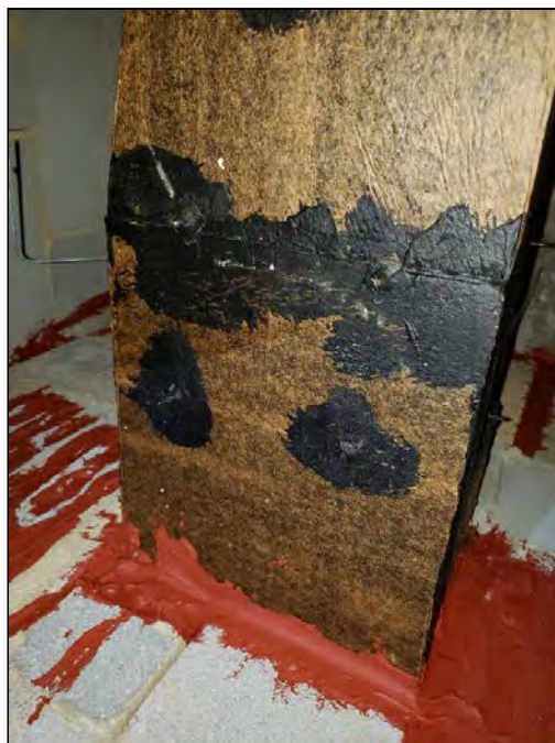
6 - Brown Fiber Duct Covering (ACM)
