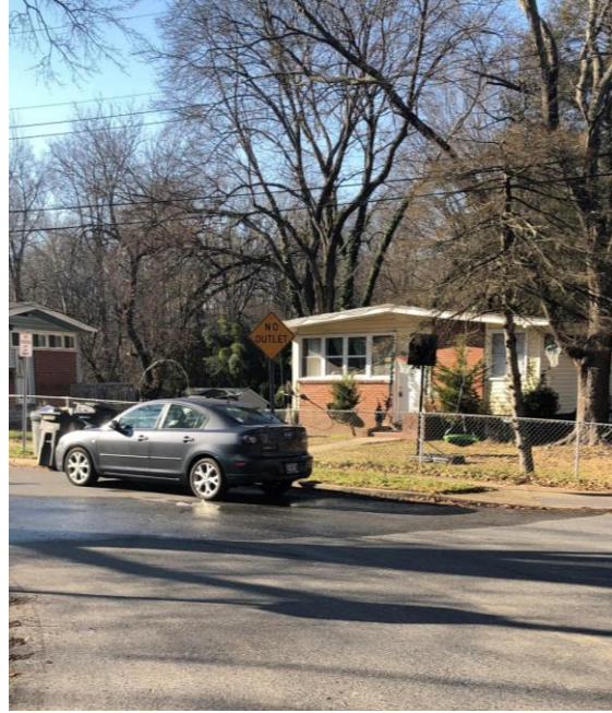
Stormwater Management/ Drainage Issue
