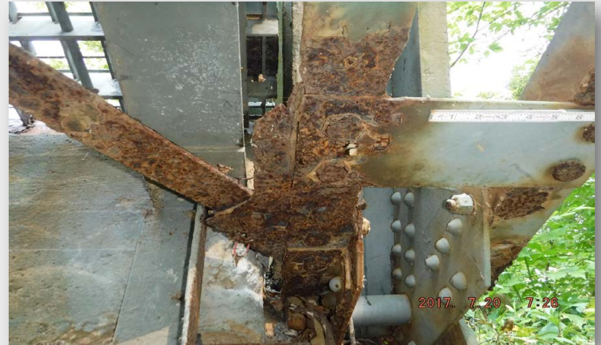
Deteriorated Bottom Steel Chords, Bottom Sway Brace and Gusset Plates
