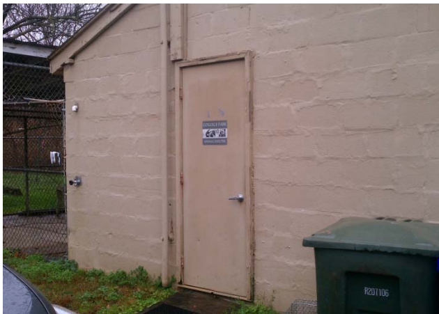
Exterior View of Entrance Door
