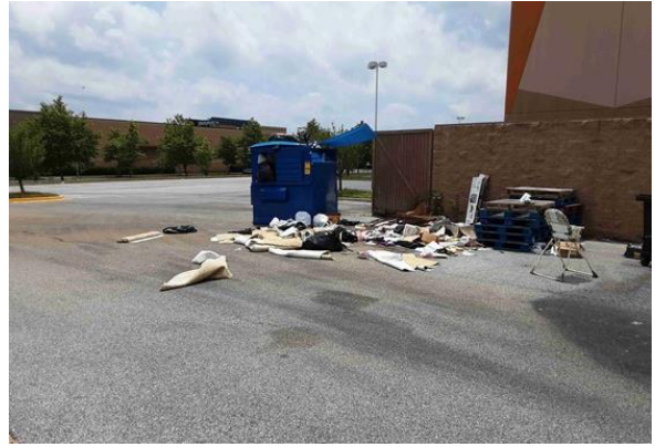
Trash and debris not disposed properly
