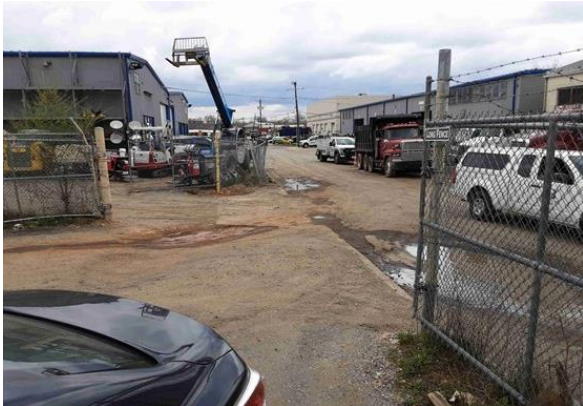
Sediment and sediment laden water entering storm drain system.
