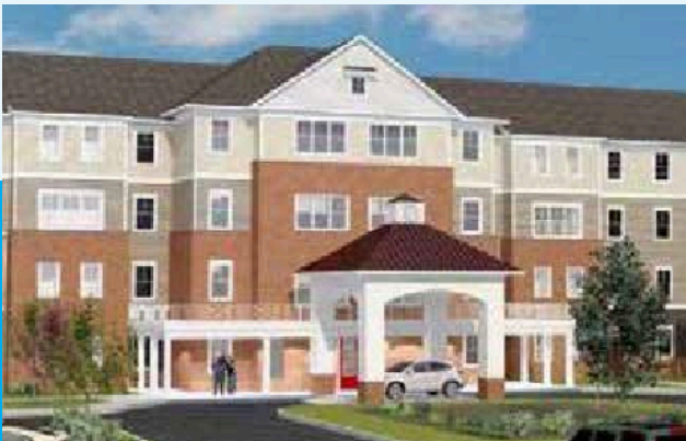
Woodyard Station Senior Building
