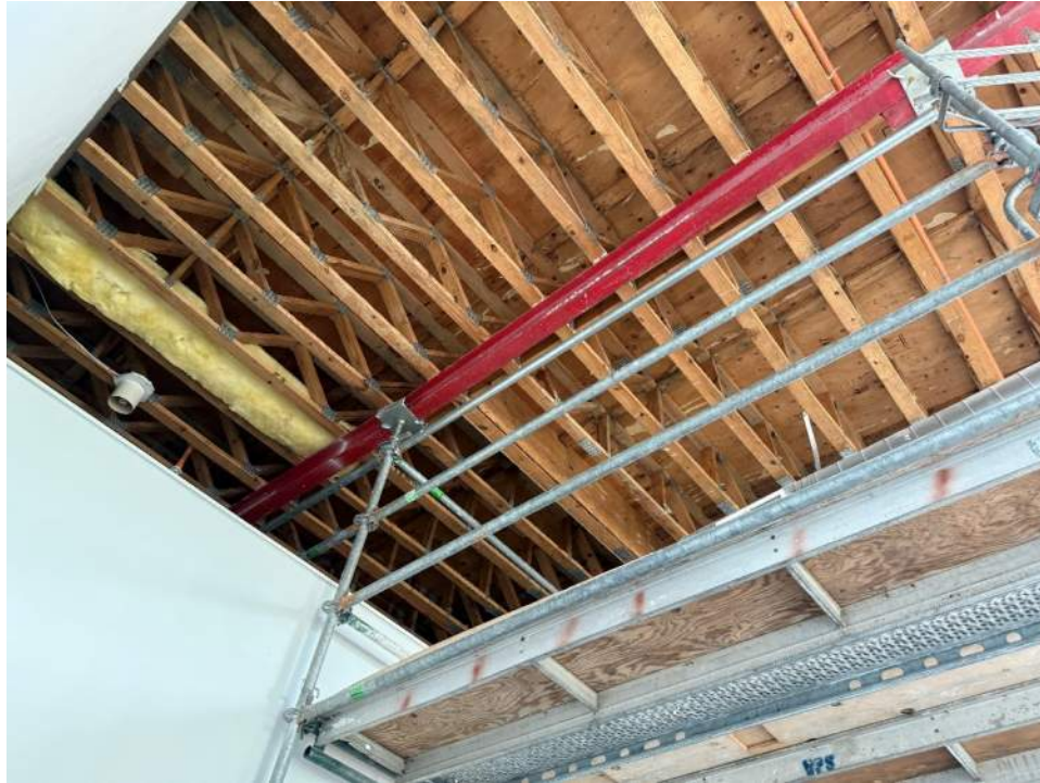
Photo 3 – Overview of Unit 202 shoring
