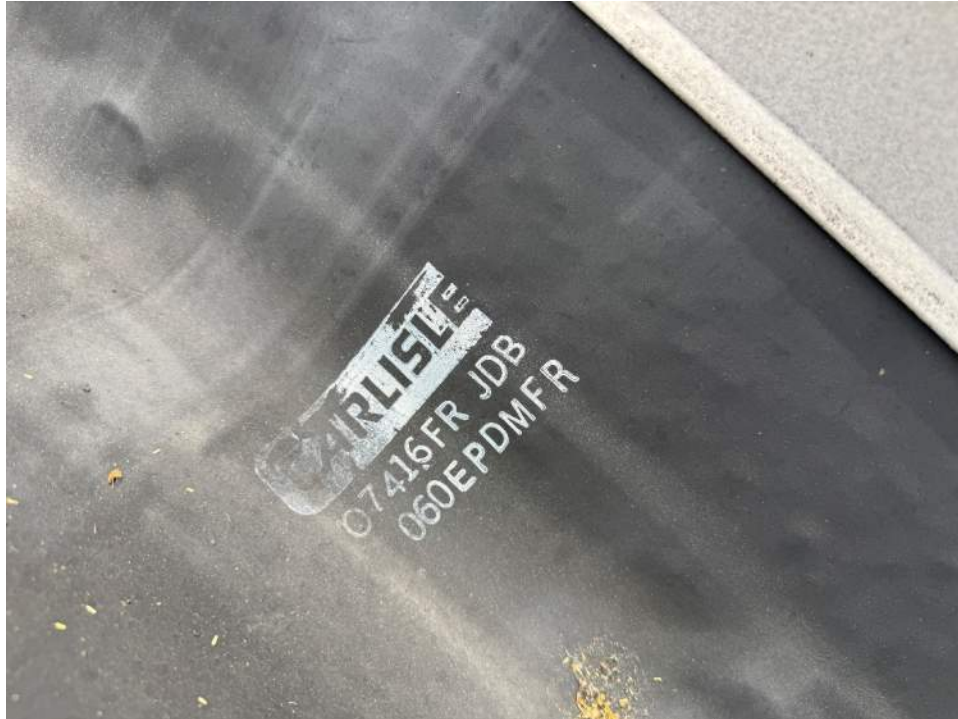
Photo 13 – Roofing system manufacturer information
