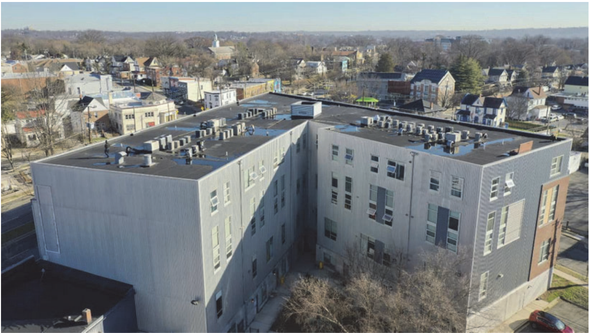
Building envelope in good condition
