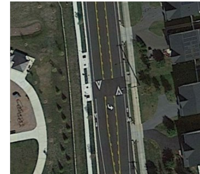
Speed Hump and Bike Lane
