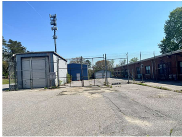
Fenced off shed buildings on site
