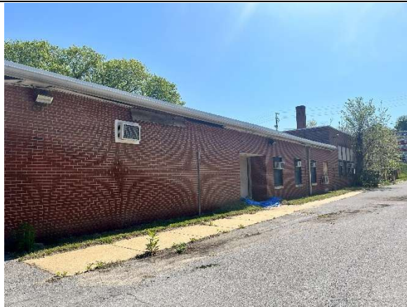
West side of vacant school building
