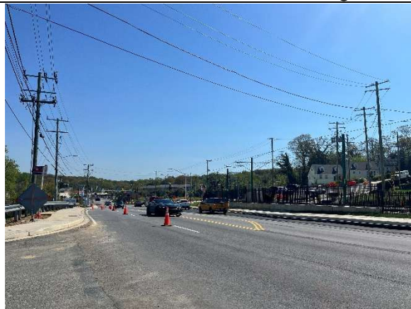
Riverdale Road facing northeast
