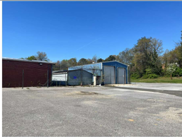
Fenced off shed buildings on site
