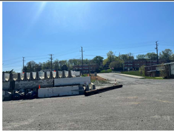
Construction materials currently stored on-site
