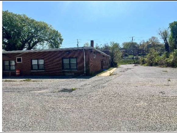
Rear and west side of vacant school building
