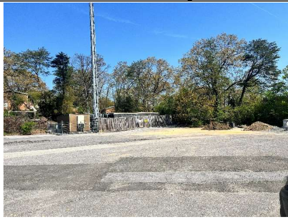
Fenced in telecommunications site
