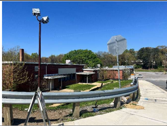
Entrance onto subject property
