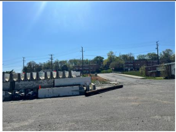
Construction materials currently stored on-site
