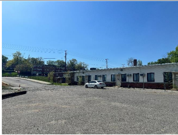
East side of vacant school building
