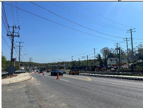
Riverdale Road facing northeast
