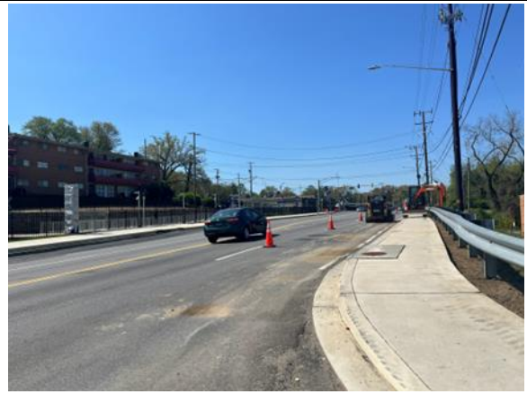
Riverdale Road facing southwest
