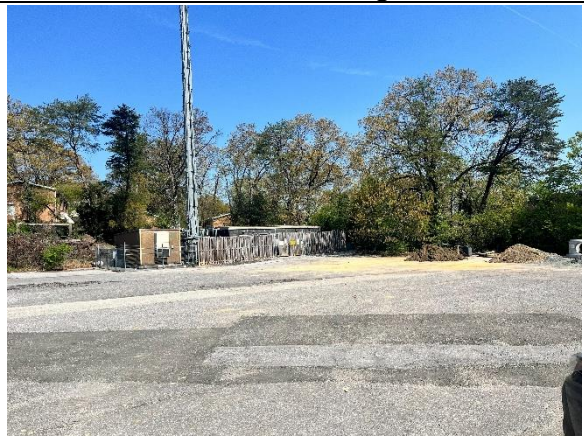
Fenced in telecommunications site
