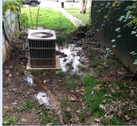
Figure 18. Saturated soil resulting from high water table (Department of the Environment).
