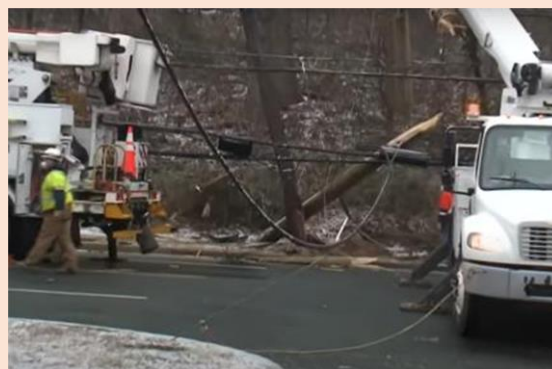
Figure 14. Downed powerlines resulting from the ice storm (WUSA9).
