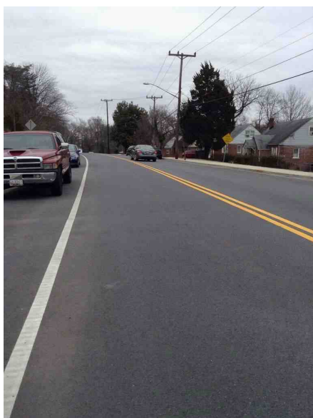
East bound view of Ray Road
