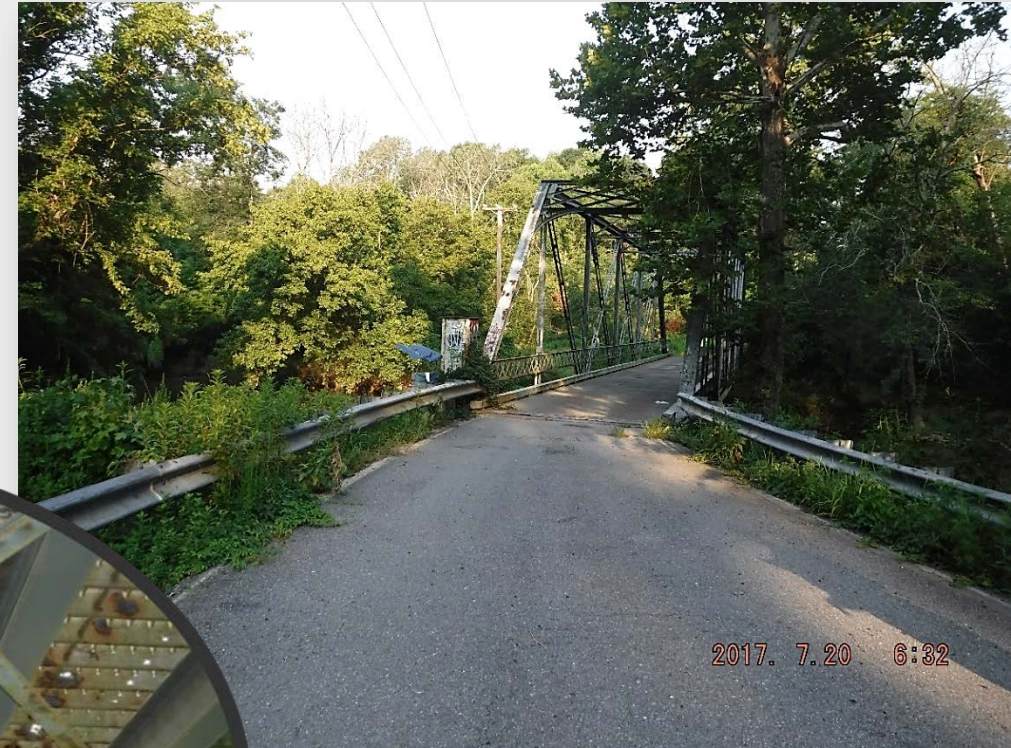
East Approach Road from Anne Arundel County side
