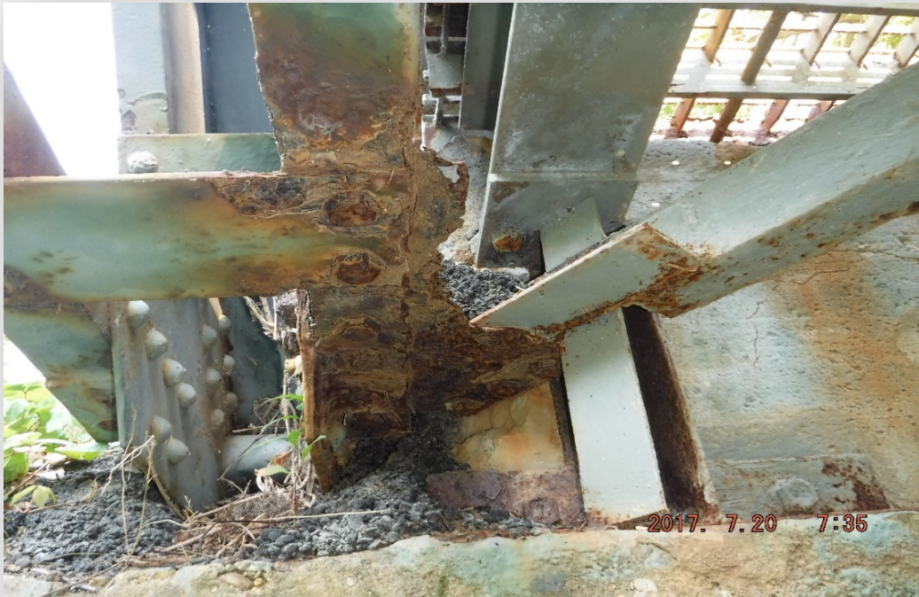
Deteriorated Bottom Steel Chords, Bottom Sway Brace and Gusset Plates
