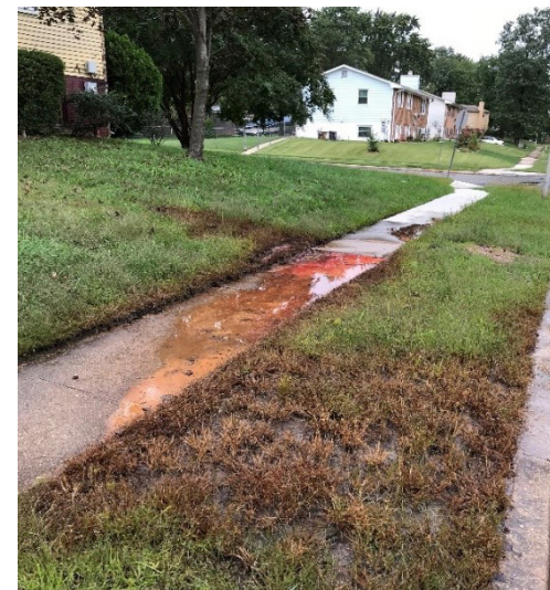
Heating oil leak.
