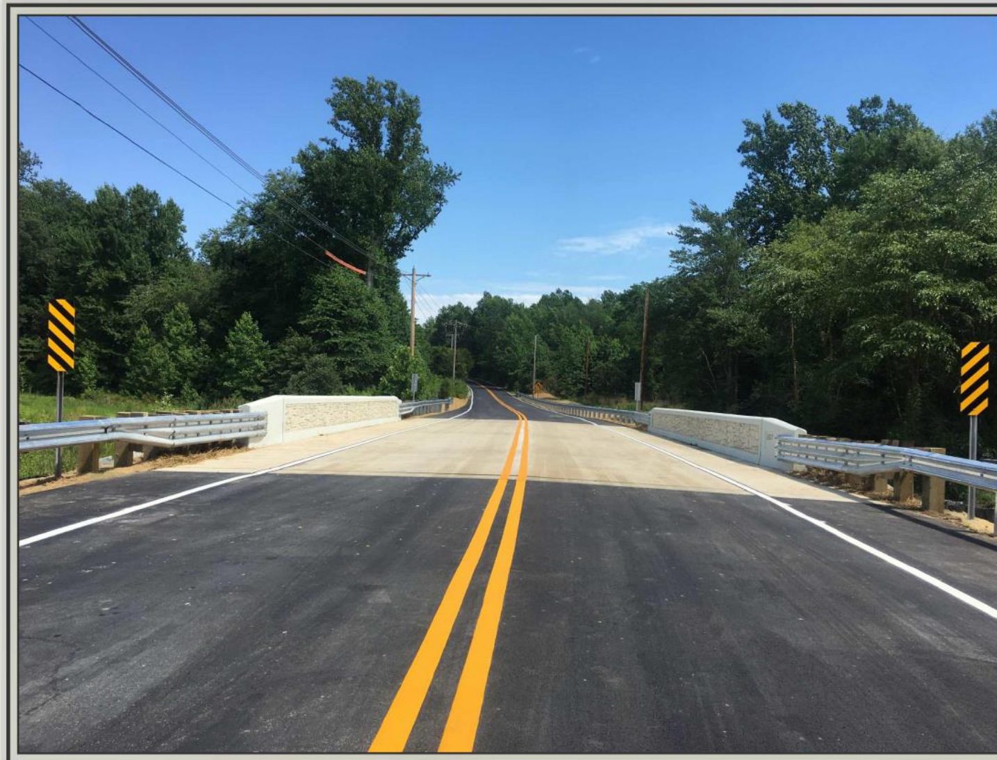
Bridge No. P-407 - Post Construction
