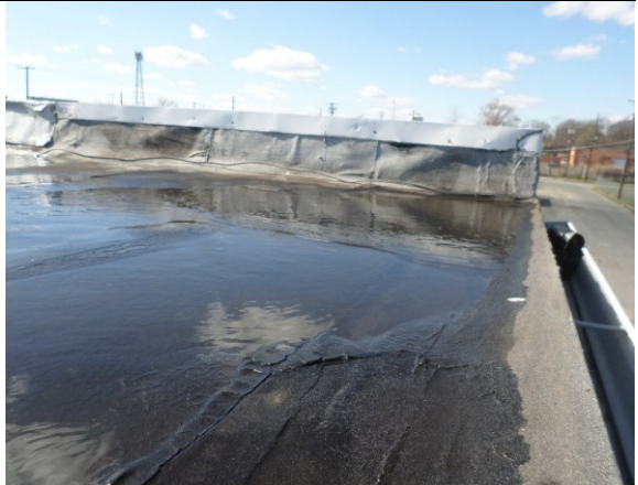
Photo #22: Rolled Roof, Roof Tar Sample Sets #13, #14 Nn-ACM
