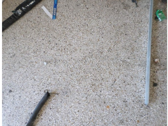
Photo #16: 4626 Main Area 12x12 Stone Pattern Tile & Mastic Sample Sets #9, #10 Non-ACM
