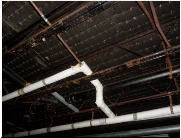
Photo #14: Basement Area Fiberglass Pipes in Basement
