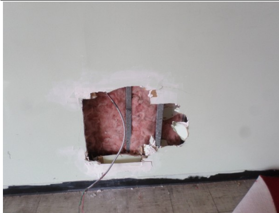
Photo #3: Typical Drywall/Joint Compound Drywall #3 Joint Compound #4 Non-ACM
