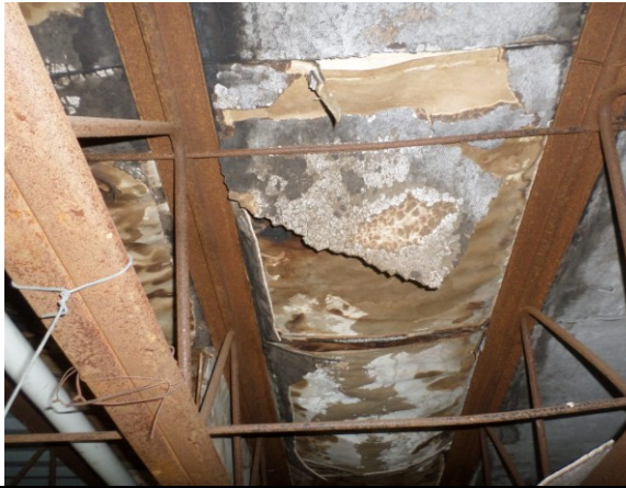
Photo #7: Typical Plaster Ceiling Sample Set #1 Non-ACM
