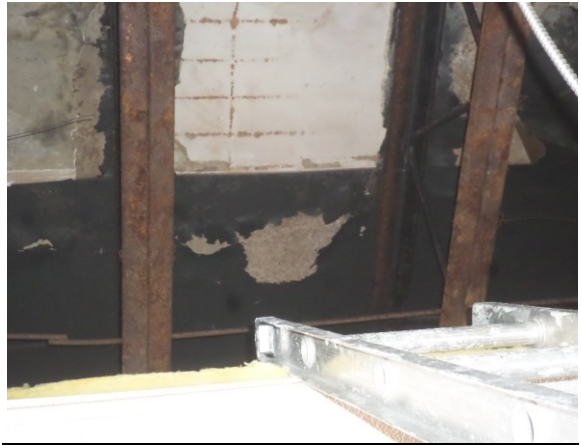
Photo #8: 4622 Roof Paper Interior Sample Set #16 Non-ACM
