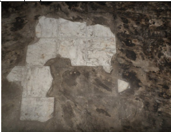
Photo #11: Basement Area 9x9 White Floor Tile and Mastic #5 and #6 Tile and Mastic ACM
