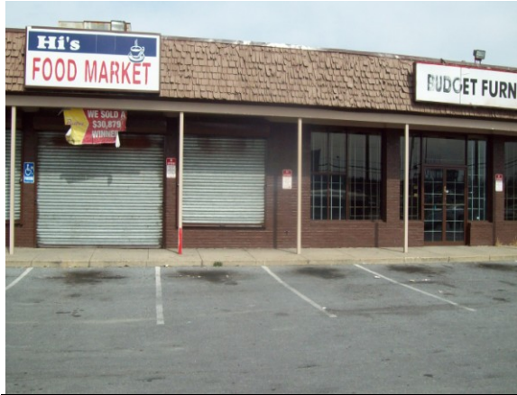
Photo #1: Front of Site
