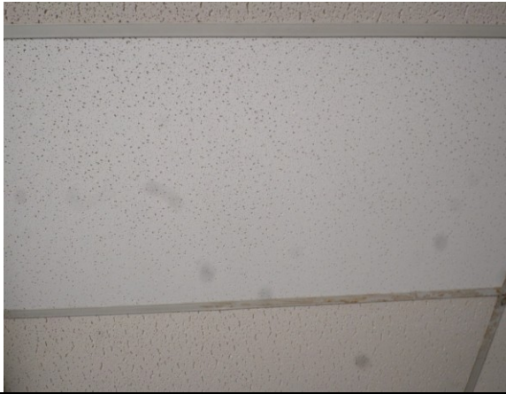
Photo #19: 4626 2x4 Pinhole Ceiling Tile Sample Set #20 Non-ACM
