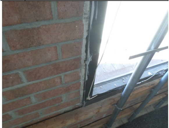
Photo #6: 4622 Interior Window Caulk Sample Set #17 Non-ACM
