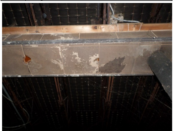
Photo #10: Basement Area 1x1 Gypsum Ceiling Tile Sample Set #21 Non-ACM
