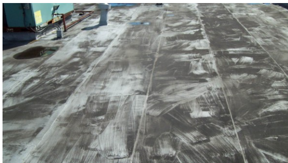
Photo #23: 4670 Roof Membrane/Tar West Side Non-ACM
