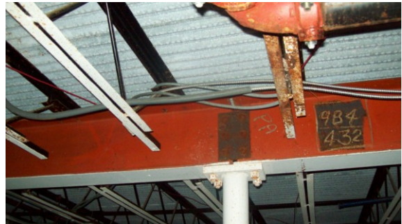
Photo #28: 4670 Plenum No Suspected ACM's
