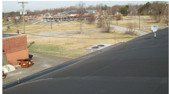
Photo #16: 4646 Roof Membrane and Insulation Samples 27A, 28A Non-ACM
