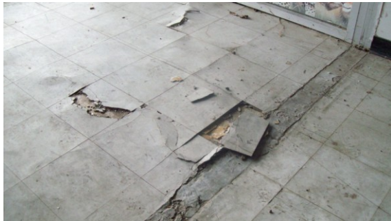
Photo #9: 4670 Foyer/Showroom Multiple Layers Tile and Flash Patch Sample Sets 11,12,13 Non-ACM
