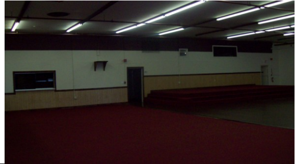
Photo #2: 4646 Interior Walls Drywall/Joint Compound/Tape Sample Sets 3, 4, 5 Non-ACM
