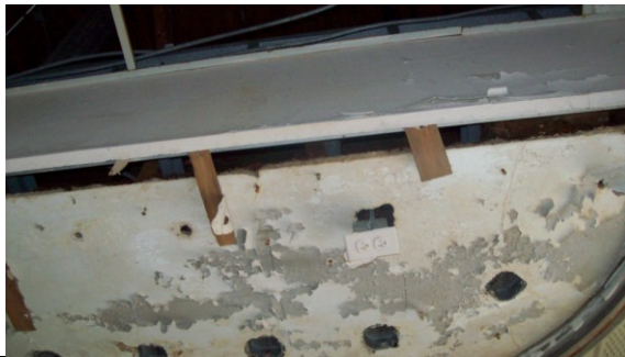
Photo #3: 4670 Soffit Plaster Sample Set 1 Non-ACM
