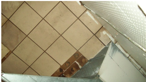
Photo #5: 4646 Hallway/Backstage Area 1'x1' Ceiling Tile and Glue Dots Sample Sets 5 and 6 Non-ACM
