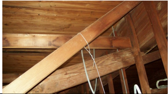
Photo #26: 4670 Plenum No Suspected ACM's
