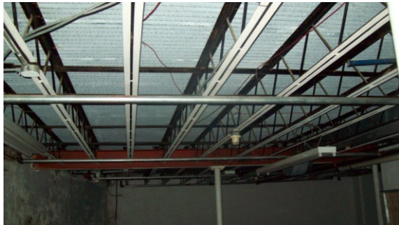
Photo #27: 4670 Plenum No Suspected ACM's
