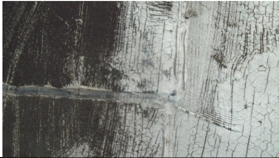
Photo #25: 4670 East Roof Membrane Sealant Sample 40A Non-ACM
