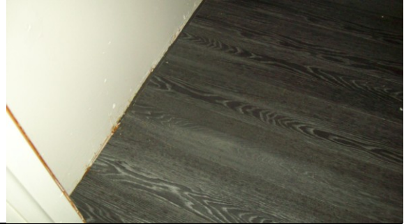
Photo #8: 4646 Mezzanine Bathroom Gray Vinyl Flooring Sample 10A Non-ACM
