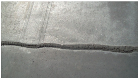
Photo #17: 4646 Roof Membrane Tar Sample 29A Non-ACM
