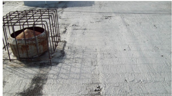
Photo #22: 4670 Roof Membrane East Side Samples 38A, 39A Non-ACM
