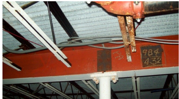
Photo #6: 4670 Plenum LBP on Beams and Support Posts
