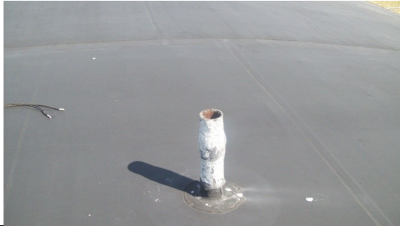
Photo #1: 4646 Roof Elevated Lead on Vent pipe
