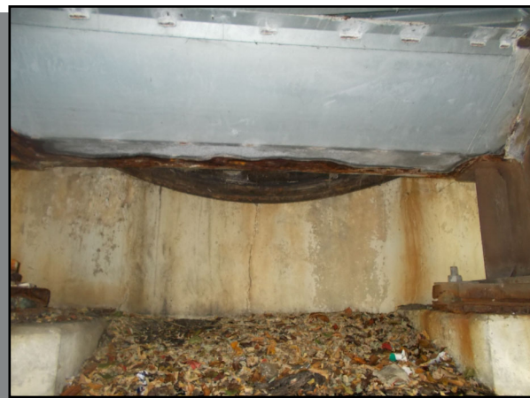
P-0198E - Detached compression seal
