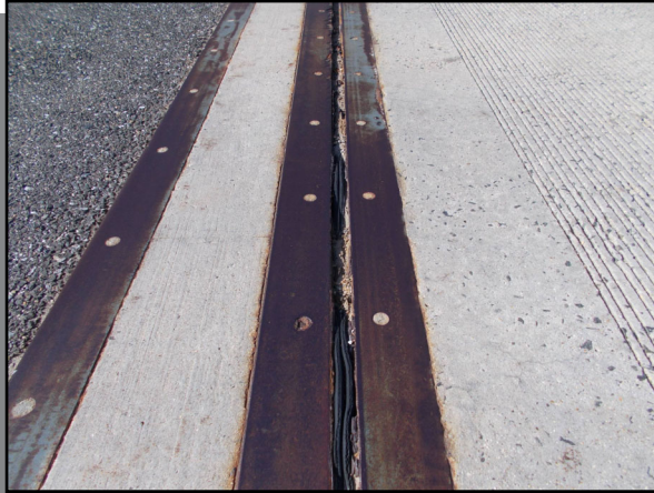
P-0490 - Tears on compression seal
