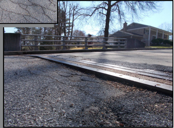
P-0579 - Settlement at the approach transition
