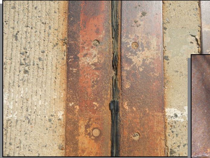
P-0596 - Tears in compression seal
