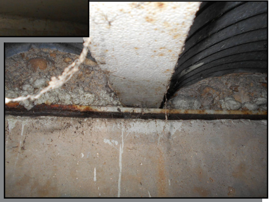
P-0220 - Rotated beam end
