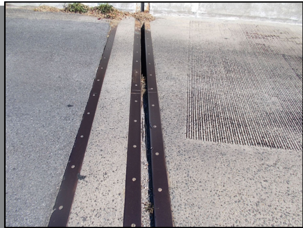
P-0198E - Depressed compression seal
