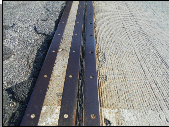
P-0484 - Tears on compression seal
