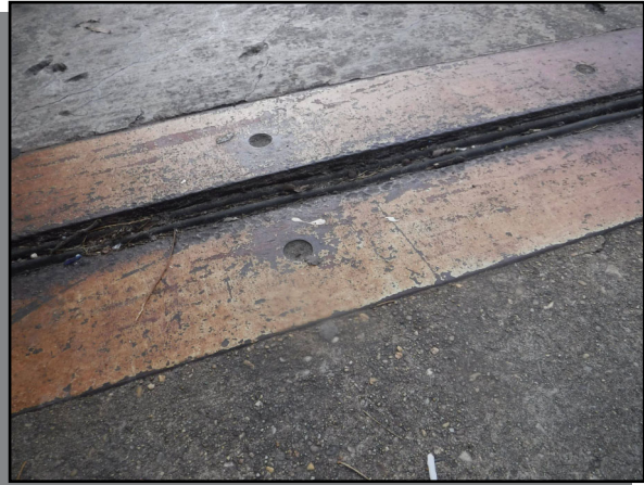
P-0273 - Tears on compression seal
