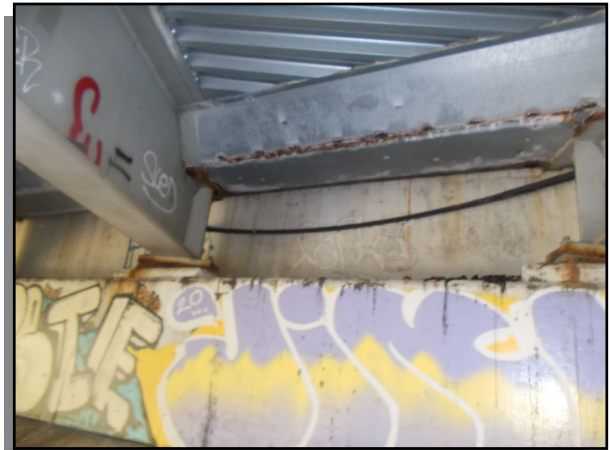
P-0169 - Detached compression seal
