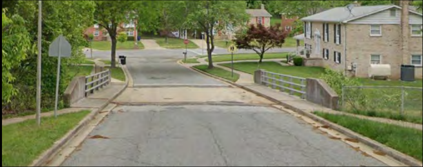
SOUTH APPROACH LOOKING NORTH
