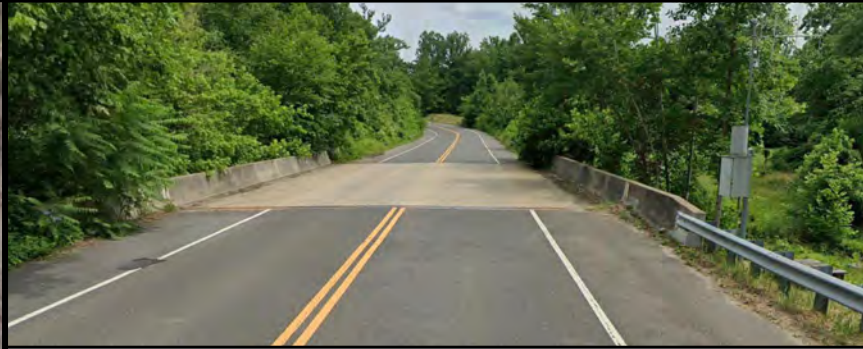
SOUTH APPROACH LOOKING NORTH
