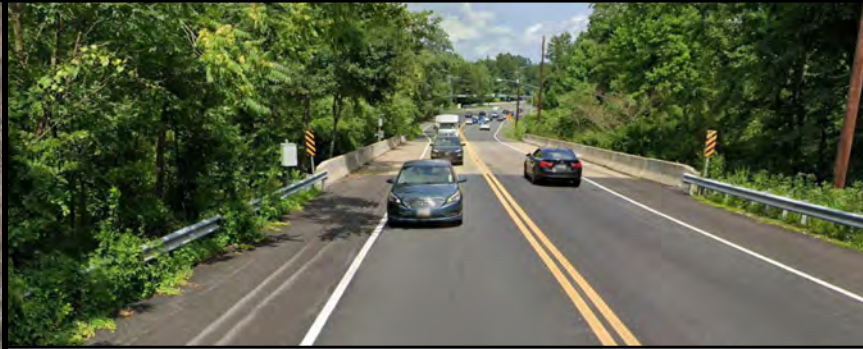
WEST APPROACH LOOKING EAST
