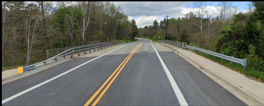
SOUTH APPROACH LOOKING NORTH
