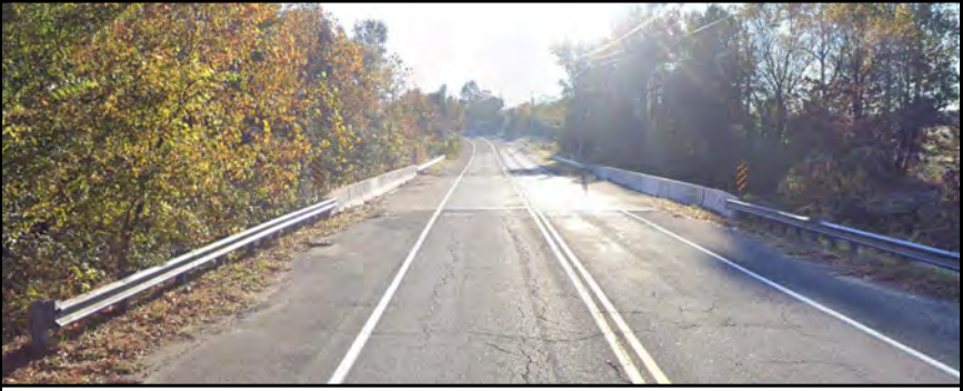
WEST APPROACH LOOKING EAST
