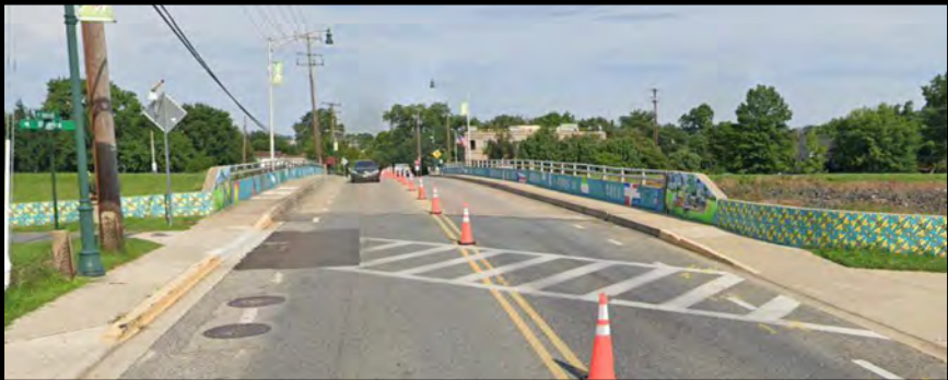
WEST APPROACH LOOKING EAST
