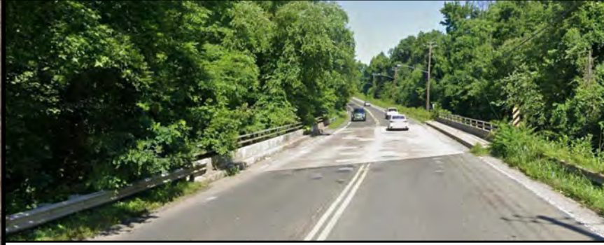
NORTH APPROACH LOOKING SOUTH
