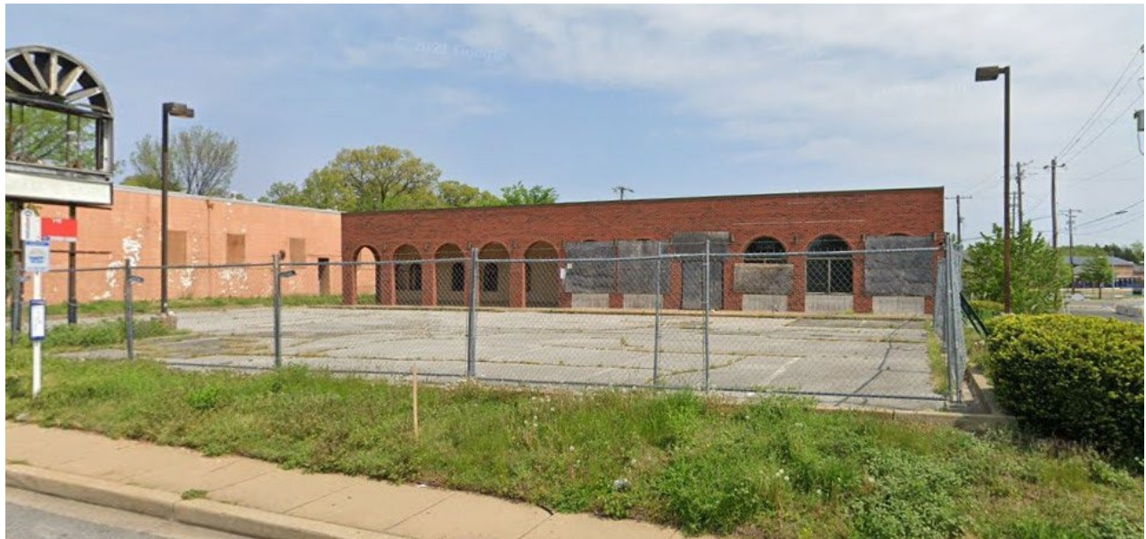
Figure 2. Street level view of 4524 Suitland Road
