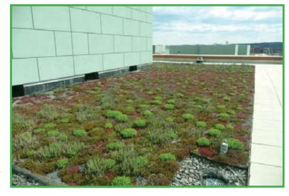
light and thin, have no public access, require little maintenance, and are suitable for residential properties. Existing roofs on porches, garages, sheds, and sunrooms are good candidates for extensive green roof retrofits. In contrast, intensive green roofs are thicker and heavier and may include shrubs and small trees planted in more than 6 inches of growing material. Intensive green roofs are often designed as accessible building amenities and are more suitable for a commercial application.
