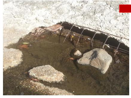
Examples of deteriorating concrete channel slabs found throughout Calverton Channel
