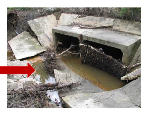
WHAT CAN HAPPEN WHEN A CONCRETE CHANNEL FAILS? Broken slabs create severe blockages which can cause system surcharges, flooding, and damage to downstream bridges, box culverts, vital storm conveyances, and transportation system structures.
