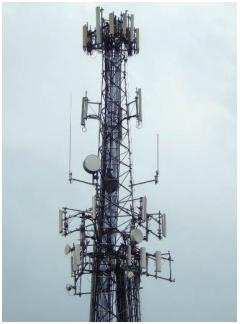
Towers include existing structures often constructed for other purposes such as those used to support electric utility transmission lines or AM radio broadcasting antennas. Towers can support multiple types of antennas for various communications purposes.
