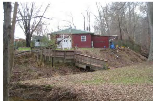
Along the west side of the property, a section of the stream bank was falling off and infringing on the garage foundation. A small footbridge that crossed the Back Branch stream was threatened.
