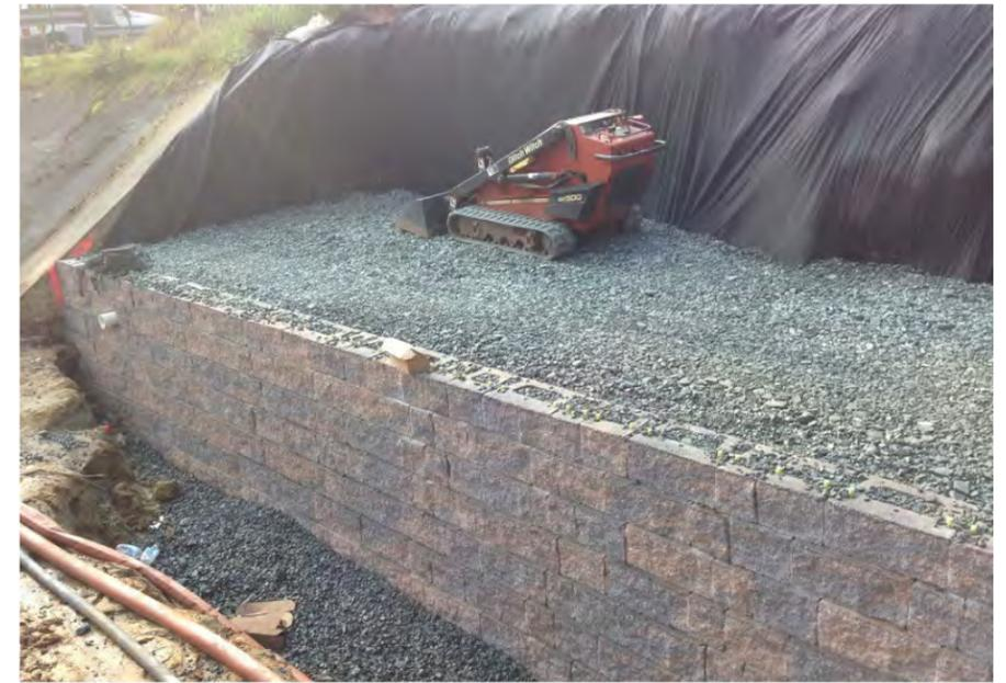
Voids in the concrete masonry units (blocks) are filled with gravel to strengthen the SRW. The gravel is then compacted to eliminate settling.
