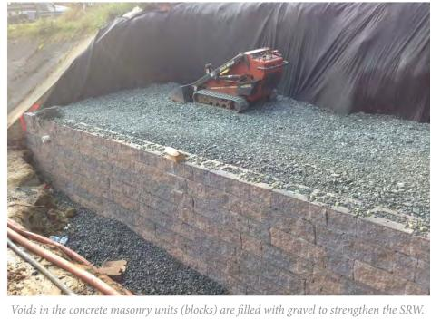
The gravel is then compacted to eliminate settling.
