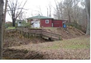
and protect the property Along the west side of the property, a section of the stream bank was falling off and infringing on the garage foundation. A small footbridge that crossed the Back Branch stream was threatened.
