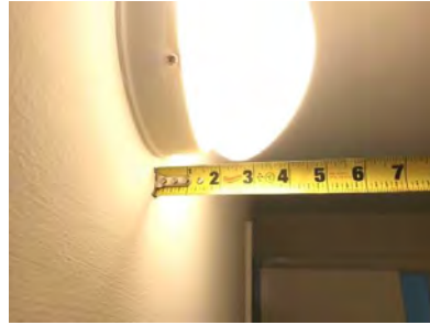
Figure 8(a) Protruding Objects Walking Parallel to a Wall
