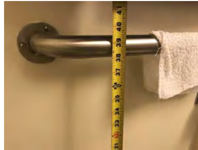
Figure 48(a) Location of Grab Bars and Controls of Adaptable Bathrooms - With Seat in Tub
