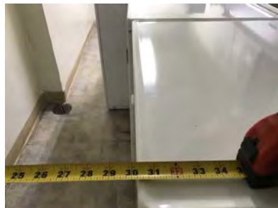
Figure 2 Minimum Clear Width for Two Wheelchairs
