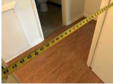
Figure 24(a) Clear Doorway Width and Depth Detail
