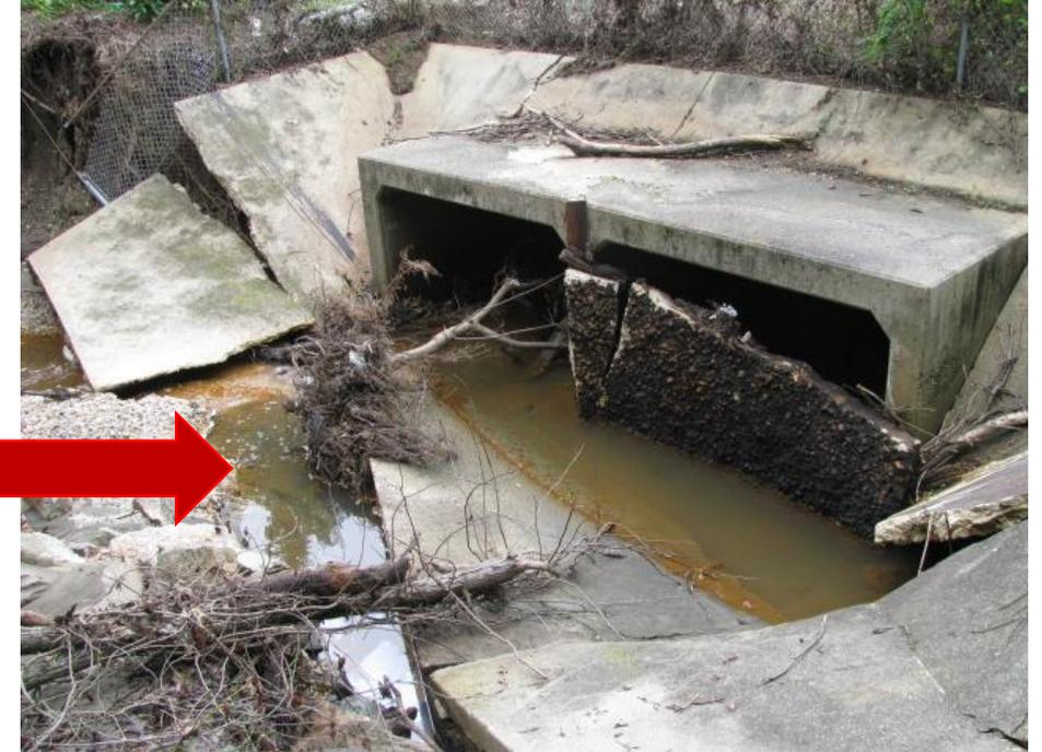
*Examples of deteriorating concrete channel slabs found throughout Calverton Channel*
